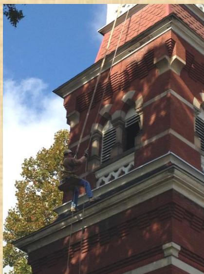
Joe Fuoco of Respond Enterprises, has begun the restoration and painting of the exterior woodwork. Joe, an experienced steeplejack, is working on both the bell tower and the lower level. Work will be completed in the Spring.
