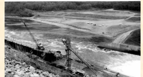
The Dam under construction
